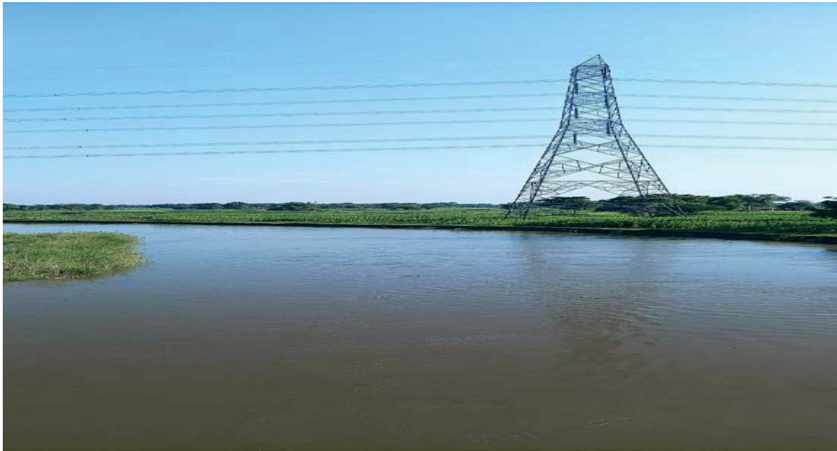
Before- Photographs of Tower no. 97
