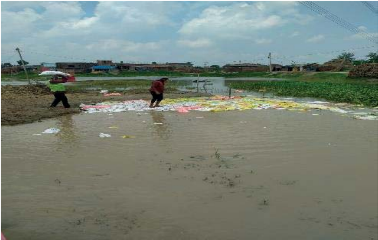
After Tower Footing Works
