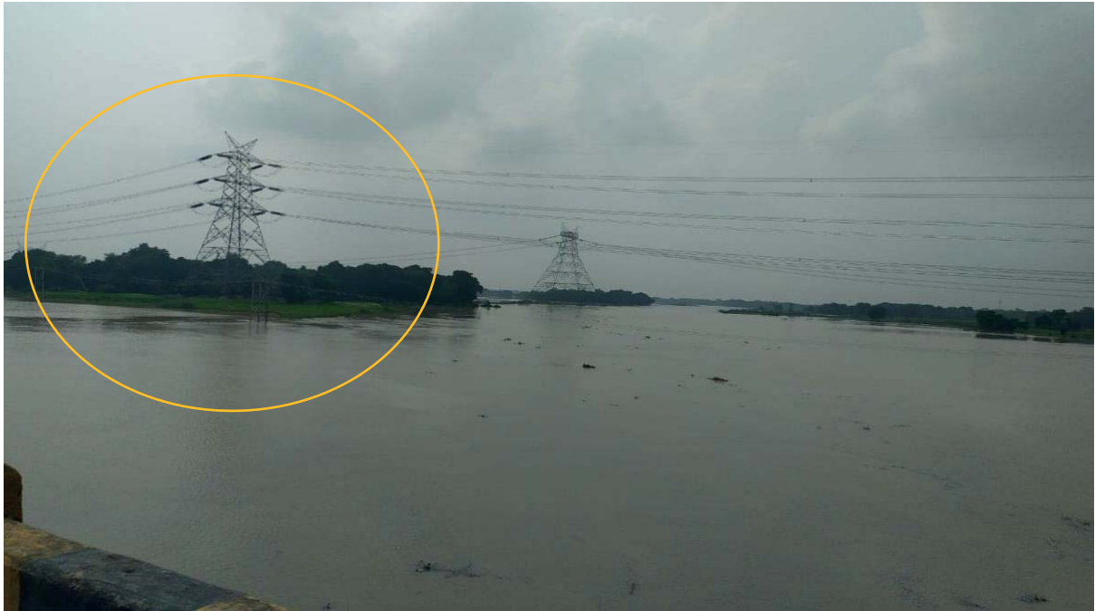
Photographs (FY2023-24) after flood situation (Pile foundation was decided)
