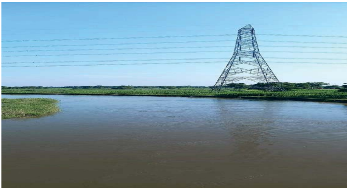
Before- Photographs of Tower no. 97
