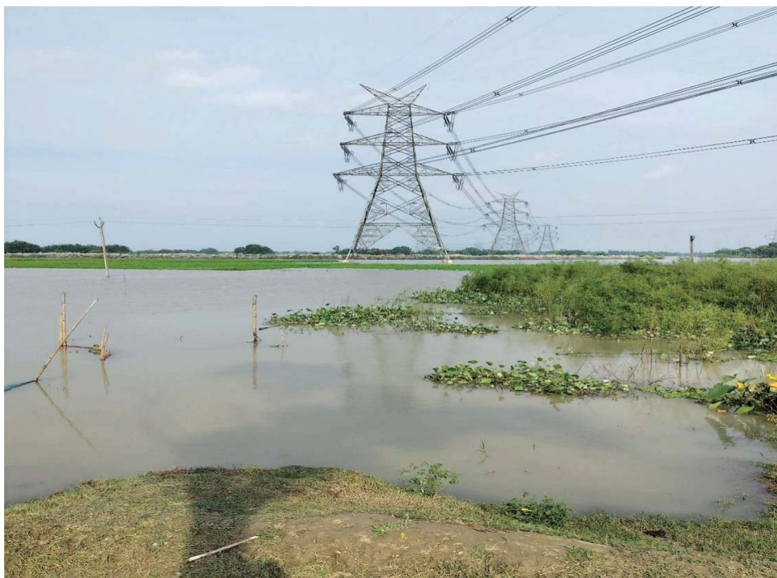
Tower 366 at the time of Floods in Parman river
