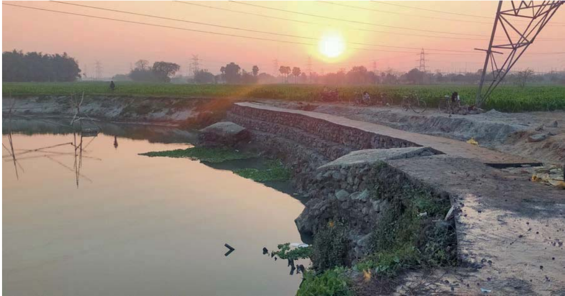
After-Photographs of surrounding area of T.No. 444, 400KV KNE-PRN(PKG#A1) under Purnea office.
