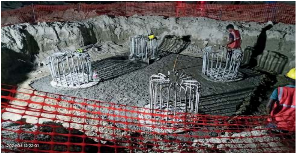
During construction of Pile Foundation
